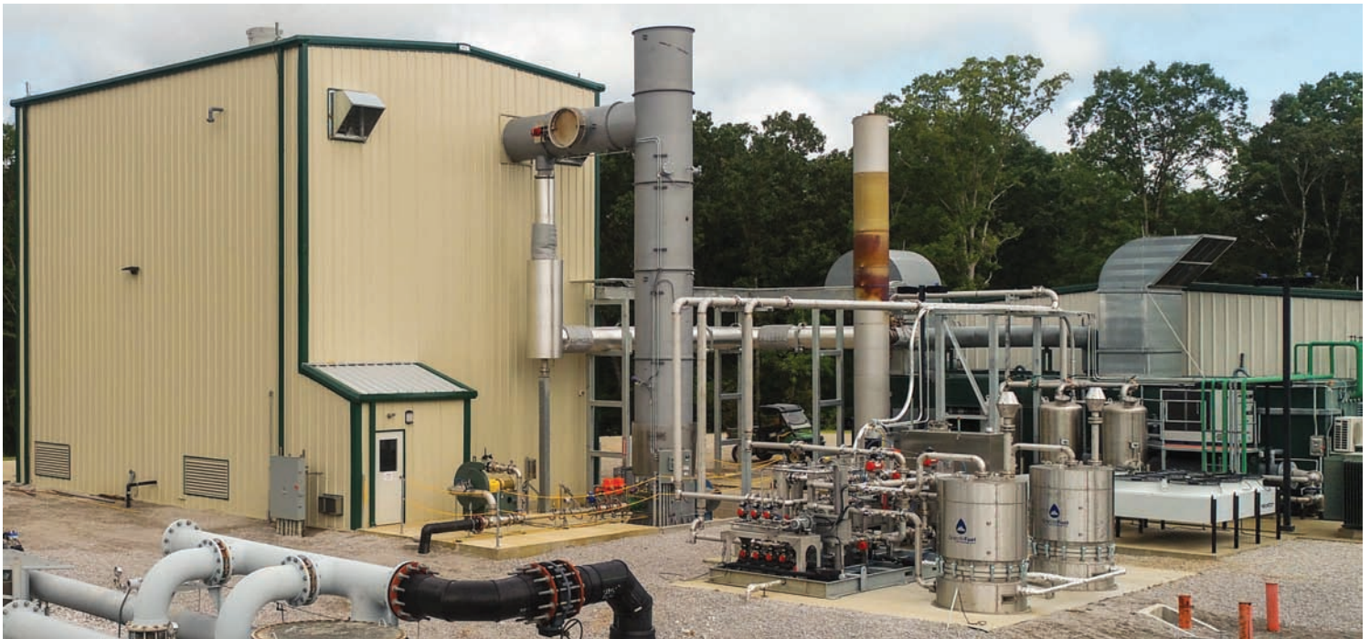
Figure 3 Hybrid configuration showing (1) integration to engine exhaust and (2) landfill gas flare.
