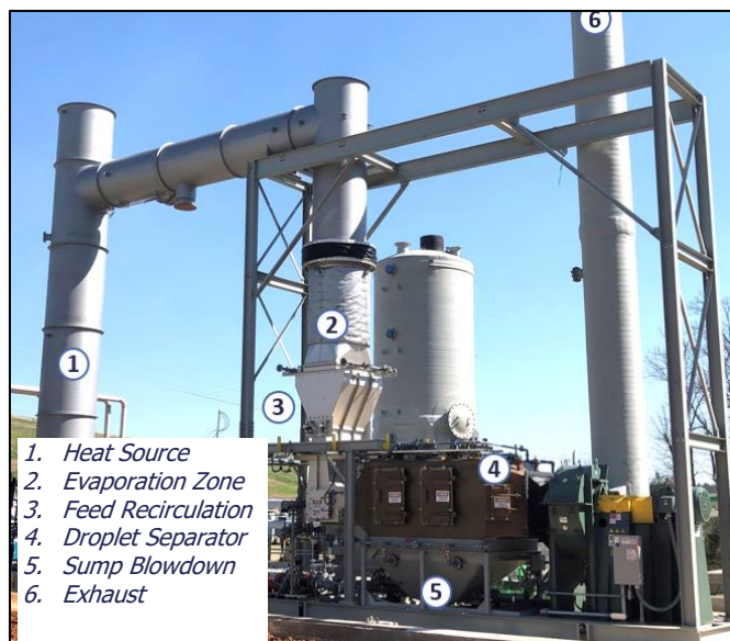
Figure 2. Heartland Concentrator shown prior to building construction
